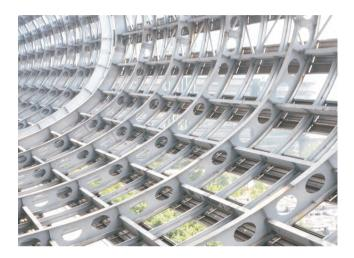
The cold rolled keel welded together to form the shield of train satiation
